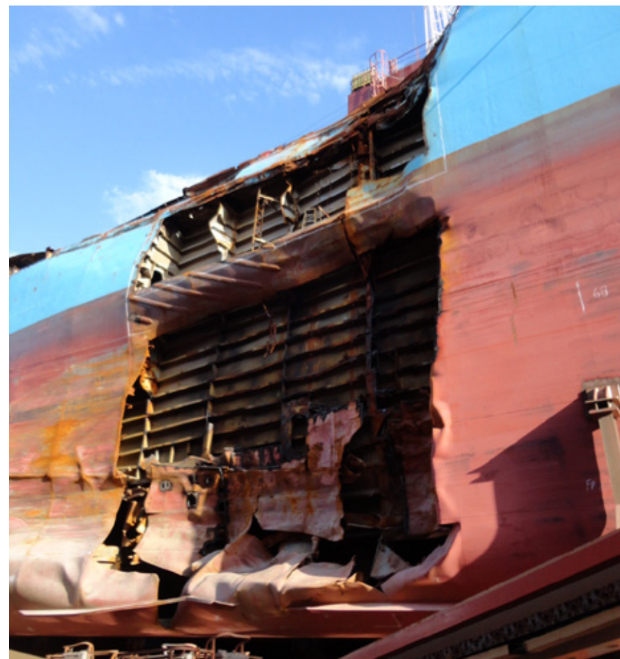
Collision, CON-DIT-CARLA MAERSK, ships damaged, 09/03/2015
